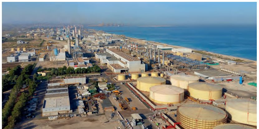
Jebel Ali Combined Cycle Power Plant with Desalination Units, Dubai, U.A.E.
