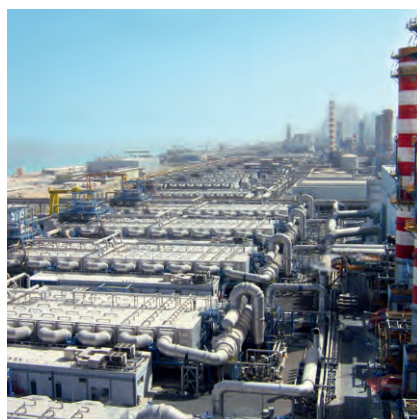
Jebel Ali Combined Cycle Power Plant with Desalination Units, Dubai, U.A.E.
