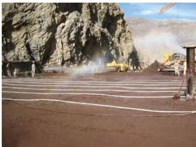
Fig. 3: Heavy equipment working on the covered cooling pipes
