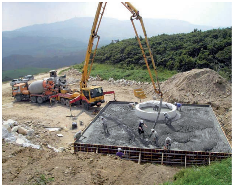
Construction in Korea
